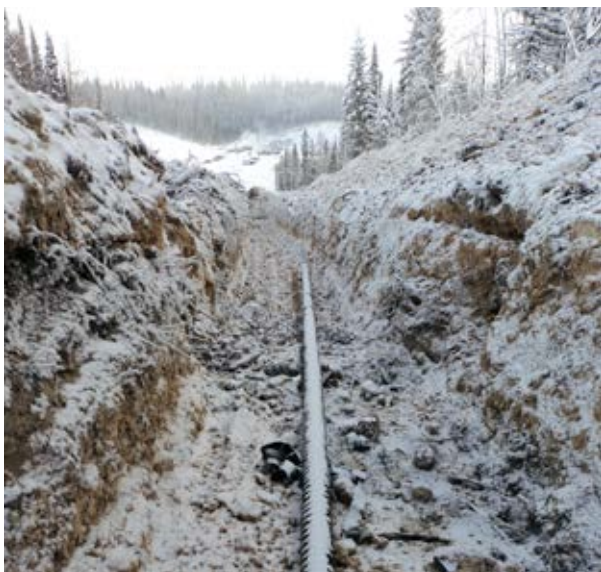
Shelton Petroleum's infield pipeline from the well to facilities
