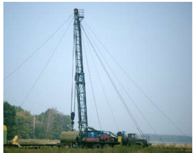
With a mobile service rig, Shelton Petroleum can resume production from old wells
