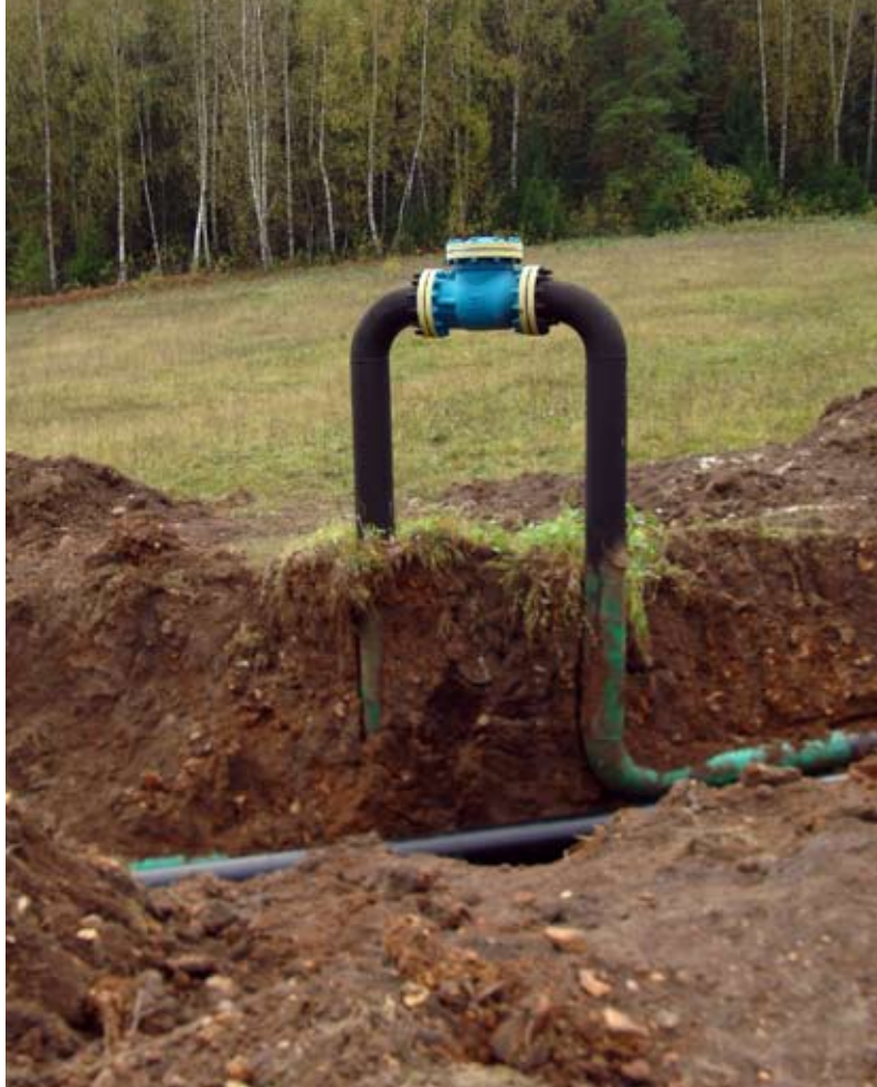
Bashneft's pipeline that goes through the license block was renovated in 2007
